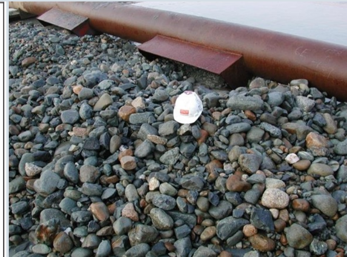
Photo above: Cobbles and boulders encountered during caisson installation, Route 6/Veterans Bridge 2007-2011
