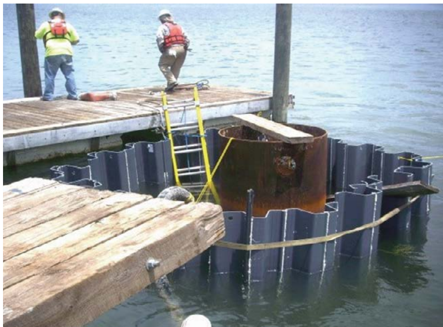
HDD Frac-out control in an emergency situation in sensitive waterway.
