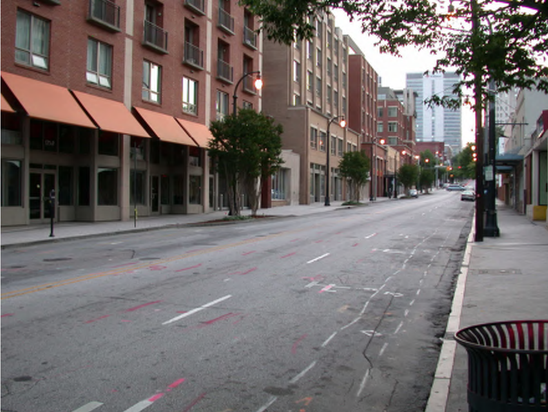
Project route at HDD entry pit location. View from east to west, and uphill.
