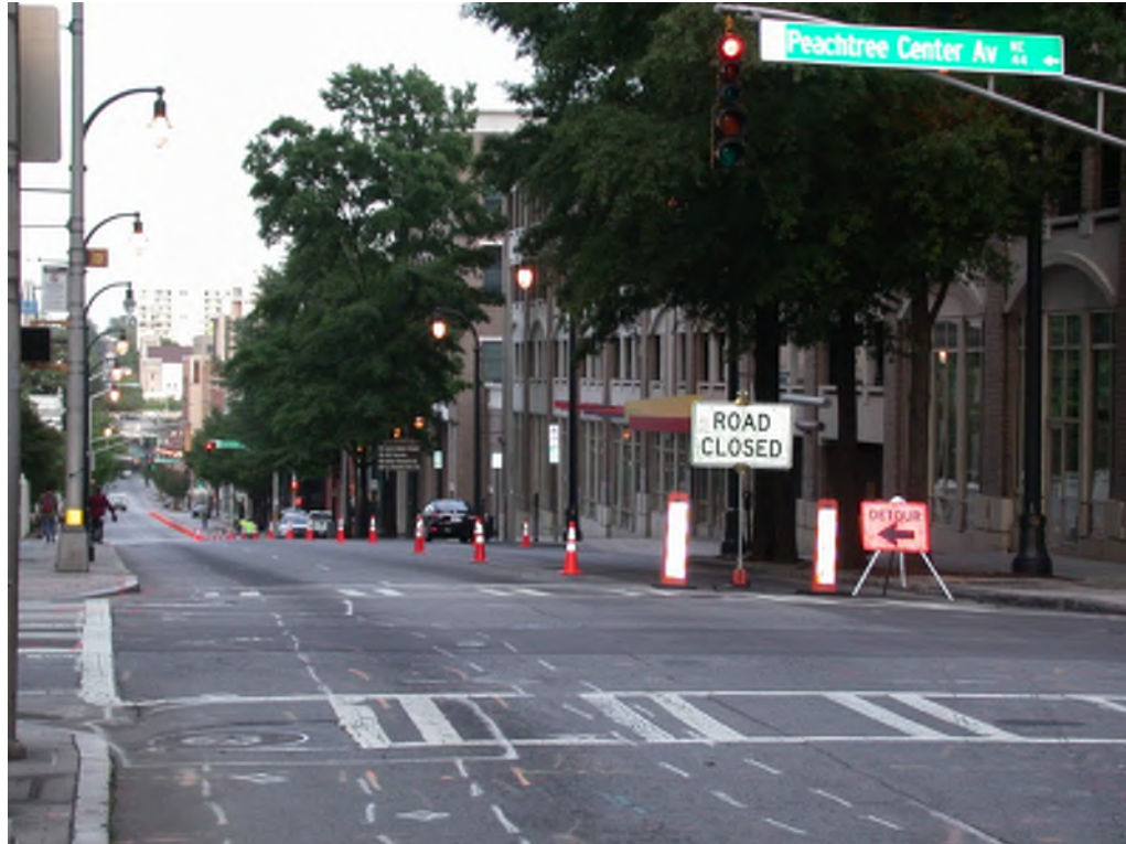
Proposed HDD route under Auburn Avenue, view to east. Note road lane closure in preparation for nighttime geophysical survey
