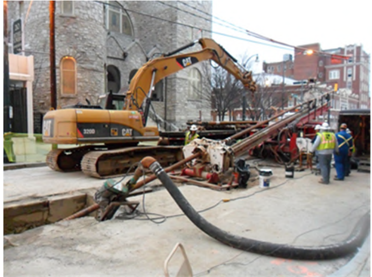
Maxi rig set up on east (entry) end near historic masonry church and beneath overhead wires
